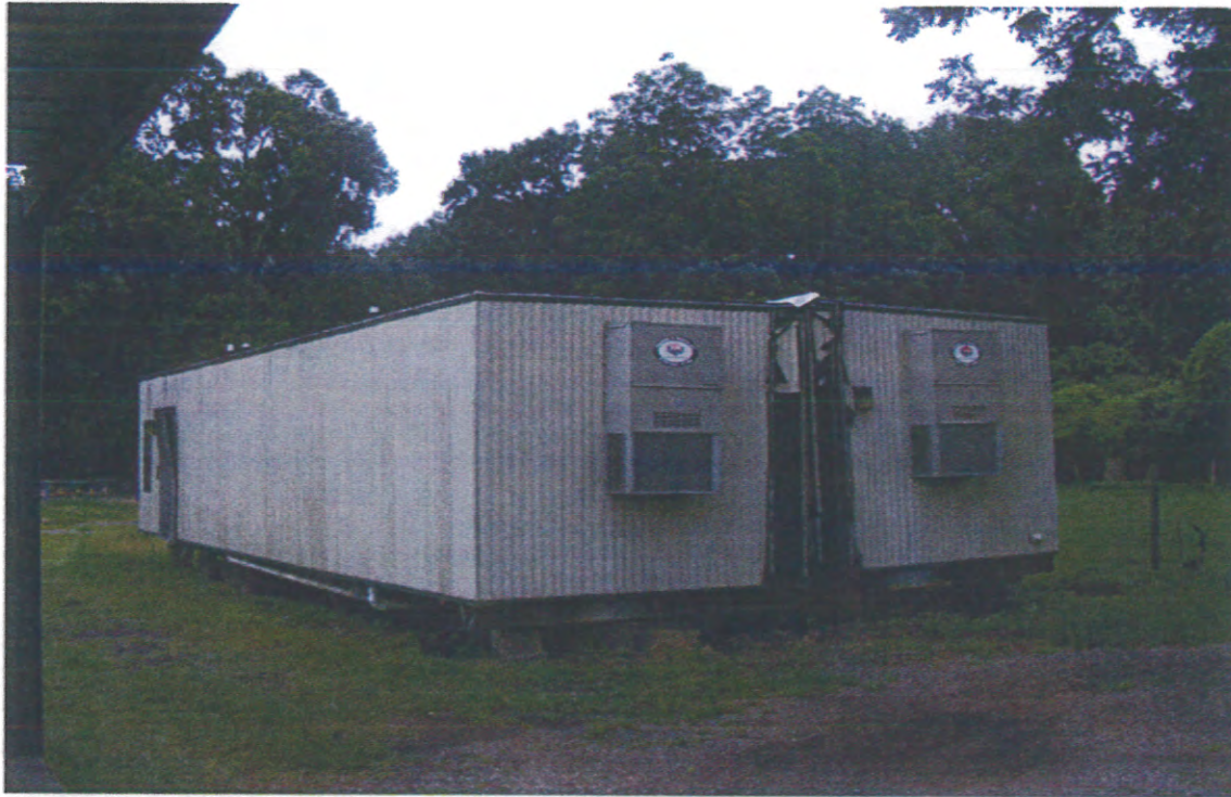
South End & West Side ↑
